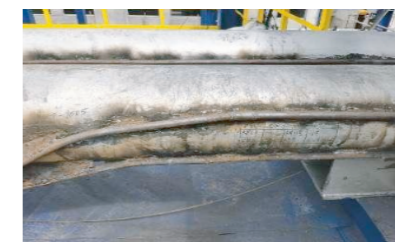
Pipeline maintenance (HTR)
